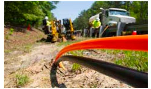
**CLASS-LEADING CYCLE TIMES.** The D40x55 S3 features a carriage speed of 188 fpm (57.3 m/min) – which is 7% faster than its predecessor, the D36x50 Series II – helping contractors install more linear feet per day.
